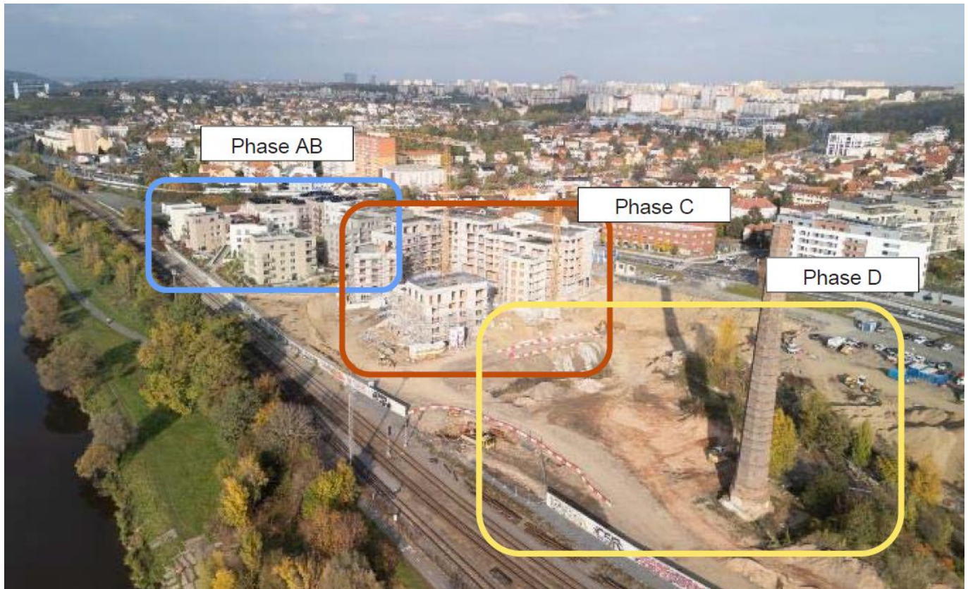
Figure 24. The MOCU project (Photo from 24.10.2024).
