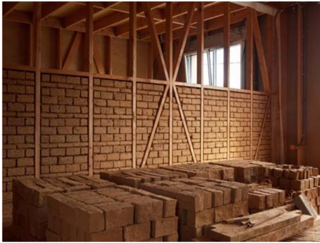
Image 9: Example of a timber-earth house (source: Germain HERRIAU, photographer)
