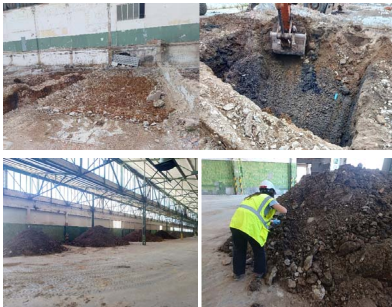
Figure 3.1-3 - Excavation and stockpiling before sieving
