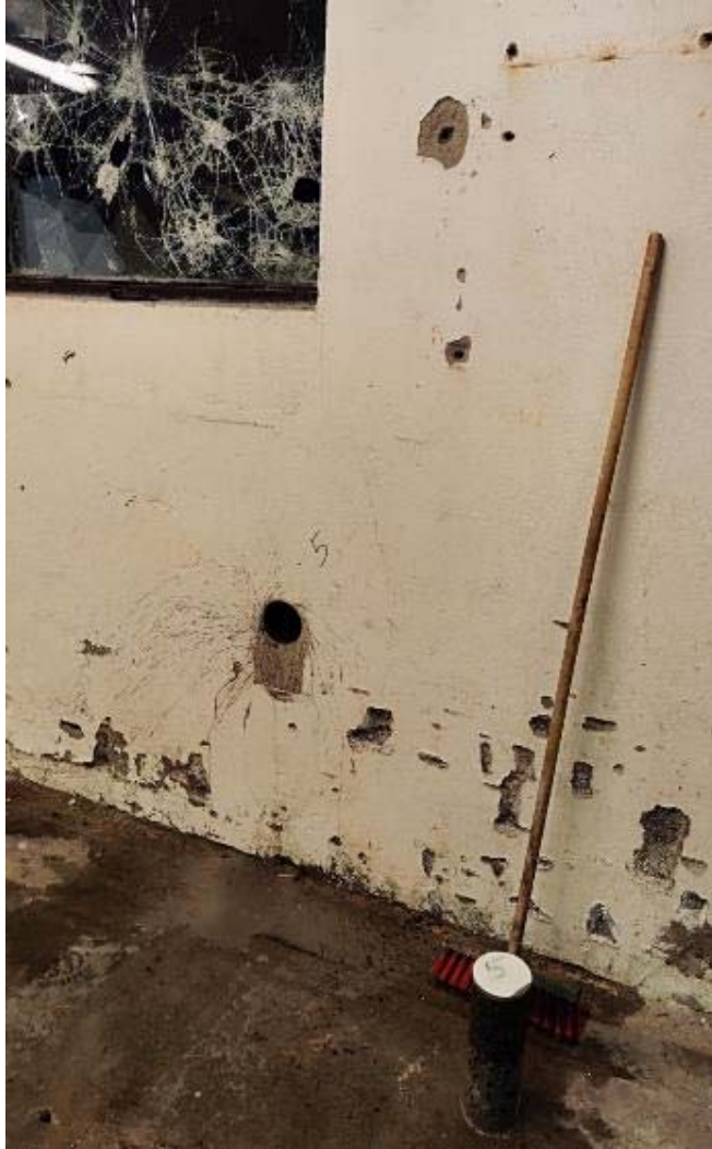
Figure 3.4-3 - Test drills for analyses of material type of individual structure parts
