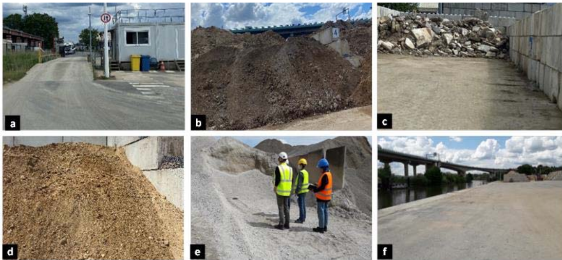
Figure18 Photograph of the Eiffage platform, a: Waste reception and control station, b, c, d: materials storage area, e, f: recycled materials storage area
